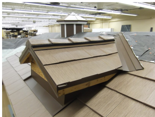
Fig. 10 captures the profile view of a dormer with a typical plastic ridge vent.
