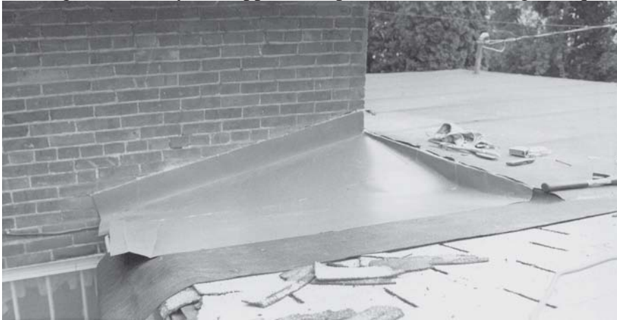
A correctly flashed blind valley.
